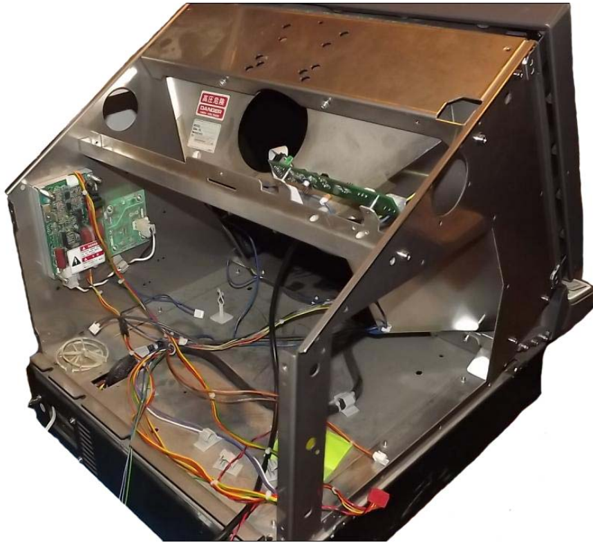
Figure 2. General view of rack with removed sweep unit and other devices
