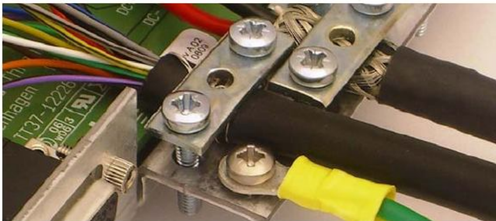
Fig. 9. Fixing the transceiver cable
