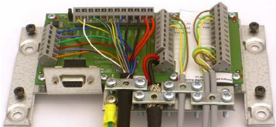
Fig. 13. Connecting the cables of the connection box with 2 alert buttons
